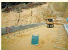
INSEM材の撒き出し転圧
