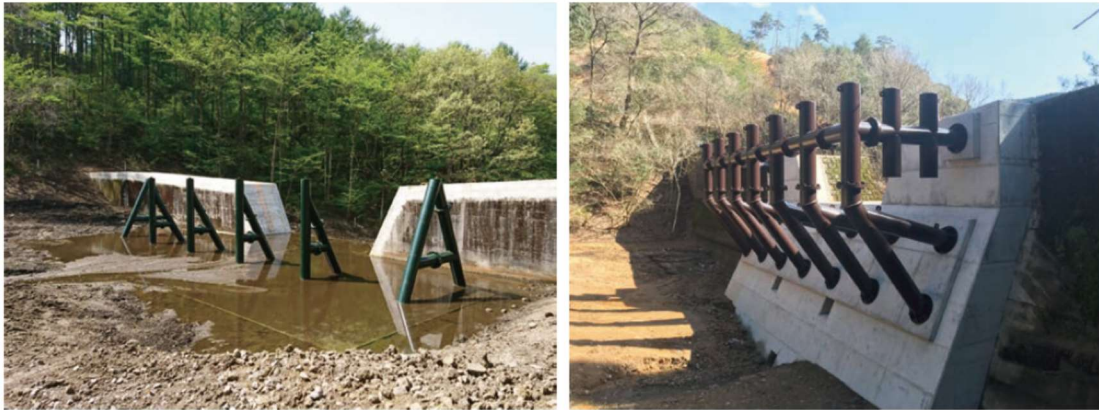
Joined rigid-frame driftwood entrappers: (left: without a margin; (right) with a margin to full sedimentation).
