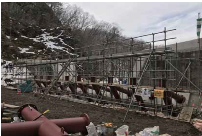
12 Lower columns installation settled
