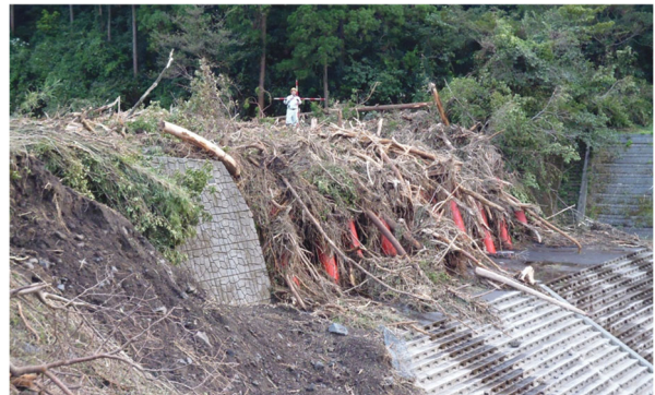
Photo 2: Driftwood entrapped with an overflow
