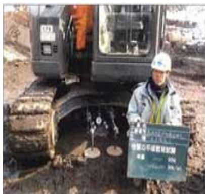
03 Plate bearing test to ensure the bearing capacity
