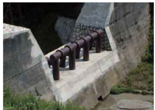
Photo-5 N type slit (cutout type)
