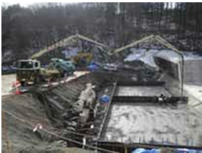
05 Concrete cast, first layer
