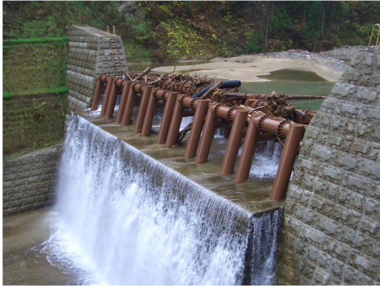
View from downstream
