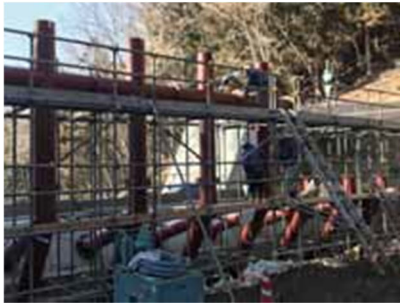
13 Center upper-part installation
