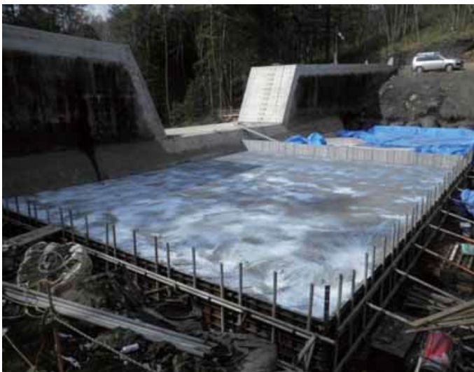
07 Completion of the 1 st layer
