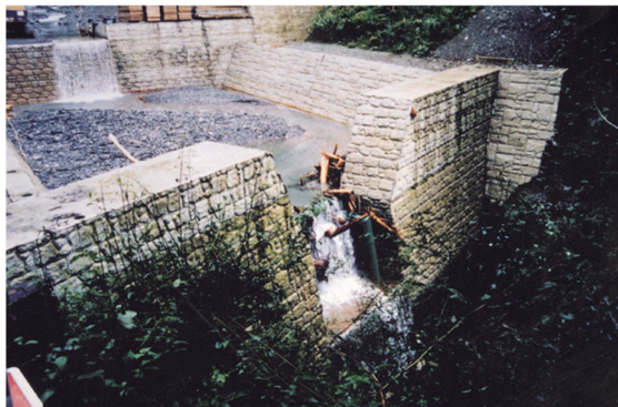
Photo 7: Driftwood entrapper joined to a secondary weir
