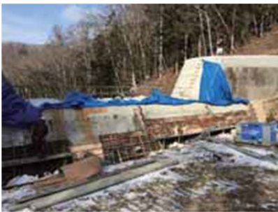
03 Formwork for filled-in concrete
