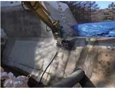
02 Chipping of existing structure
