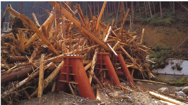
Photo 1: Driftwood entrapped without overflow
