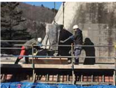
04 Casting filled-in concrete
