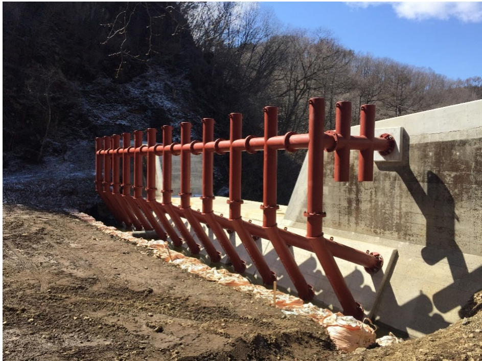
Photo 6: With margin to the full-sediment level: Futamatasawa No. 2 Sabo Dam (MLIT Tone River System Sabo Office)
