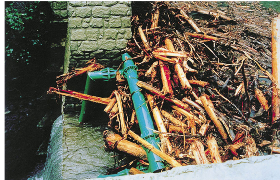
Photo 7: Driftwood entrapper joined to a secondary weir
