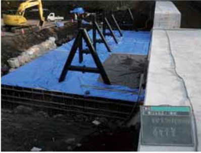
13 Concrete cured with plastic sheet
