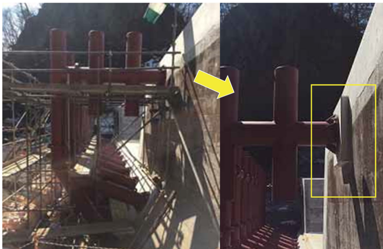
16 Edge modified concrete installation
