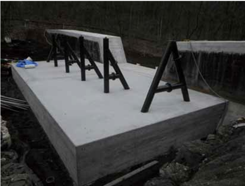
14 Concrete casting completed
