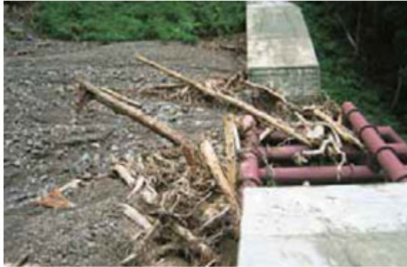
Photo 2 Steel open type Sabo dams capturing driftwood
