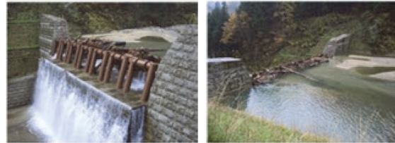
Fig.2 Sediment and driftwood capture at partially hydraulically consecutive sabo dam
